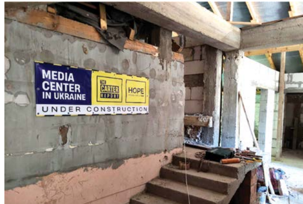
The Carter Report Hope Media Center in Western Ukraine is being built to reach people in Ukraine and Eastern Europe.
